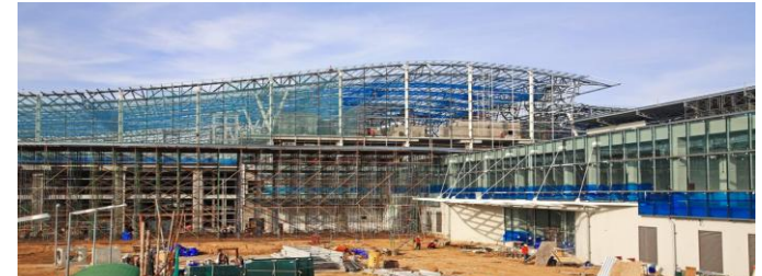
Zeghamra International Airport Development
